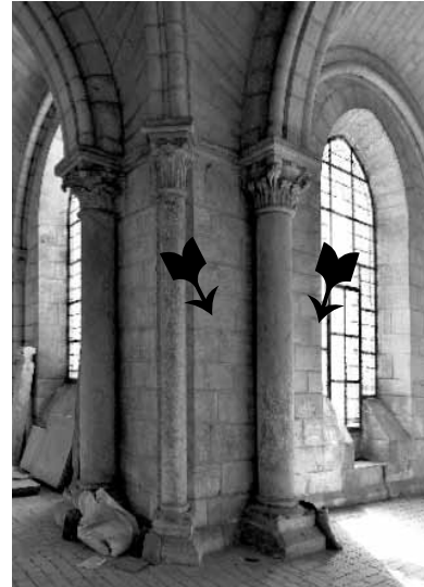
Broken coursing behind the Es2w doubleau shaft.
