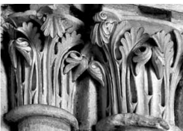
François 2 capitals in EN6 pier
