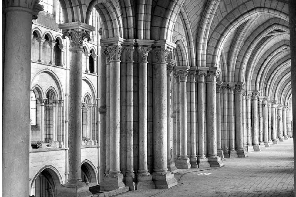
Arrangement of the nine capitals on a pier
