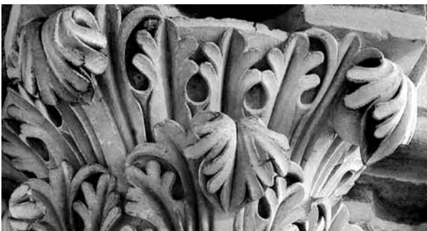
Philibert triple-leaf arrangement on the EN2w pier
