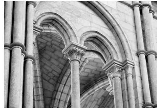
Laon cathedral, south gallery showing the central shaft between the piers, and below a plan of a typical wall pier with five shafts and an arcade pier with nine, in which three support the arches of the opening into the choir while the inner three support the ribs and doubleau of the gallery.
