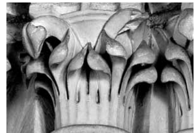
Lazare on adjoining pier NE3
